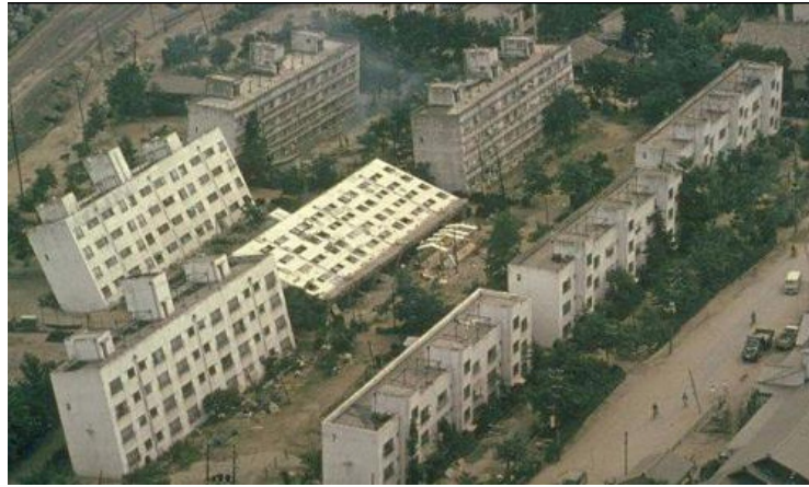
Figure 3-21: Apartment buildings after the 1964 Niigata, Japan earthquake.
